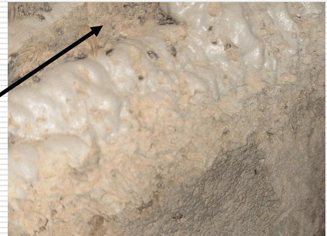
NOTE: If producer can't control their beetles, it is questionable if spray polyurethane foam insulation is the right choice for enclosing their curtain-sided houses
