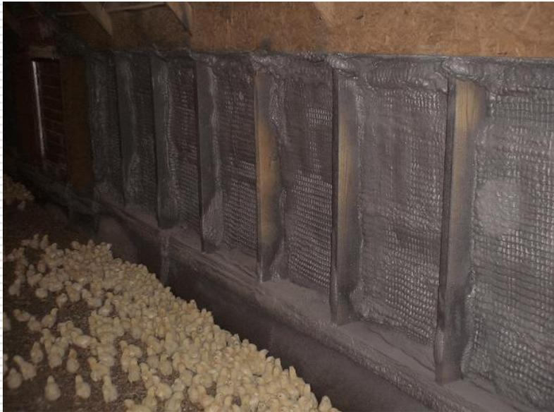
**Curtain sprayed with polyurethane insulation**
